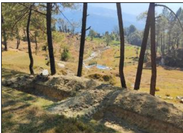
Construction of trenches and gabions in Kamyaraula project, Almora district, Uttarakhand
