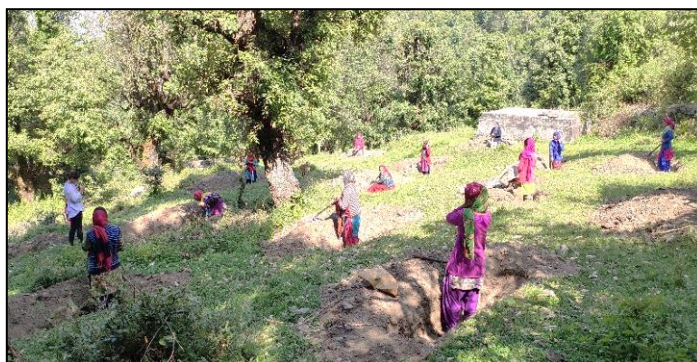
Trenches excavation work in Bajwad village
