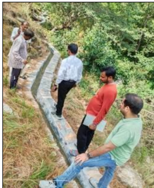
Construction and repair of Irrigation Guhl in Kamyaraula project
