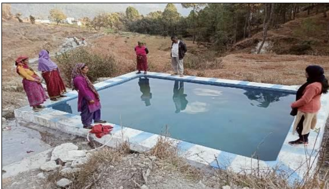
Construction of storage tank for irrigation in Khirganga project, Kapkot, Bageshwar
