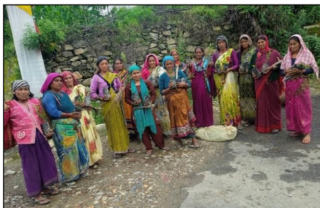
Plantation work at Haskoti village
